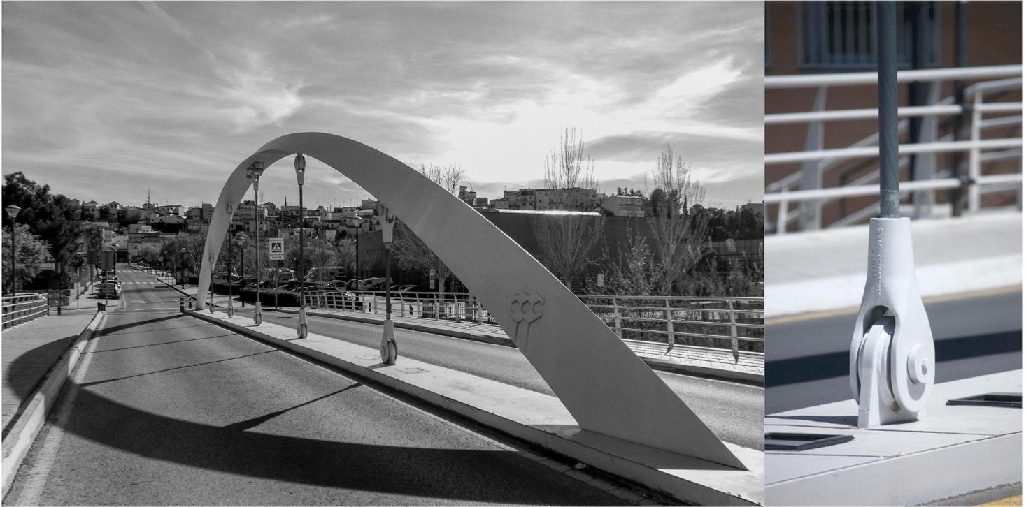
The structure of the project consists of a composite deck, a steel arch with a single span of 31.00 m between supports, five closed galvanized steel cables and load-supporting reinforced concrete abutments. The total width of the structure is 14.00 m, divided into a central part of 9.00 m for road traffic and two 2.50 m lateral parts for pedestrian use.
